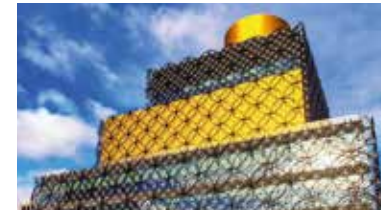
Connection of facade lighting devices at Birmingham library (UK). Series TH405/TH631.
